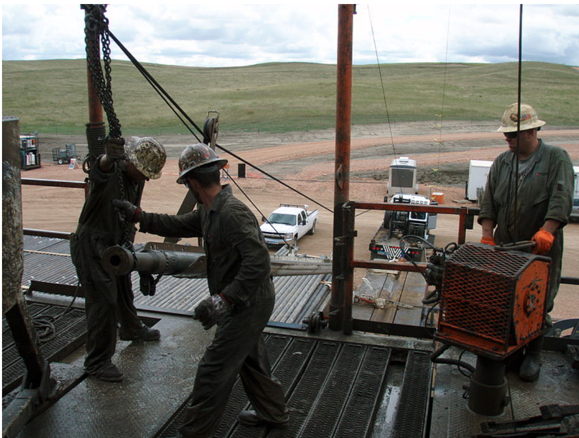
Figure 2-6. Pulling drill pipe onto the drilling platform.
