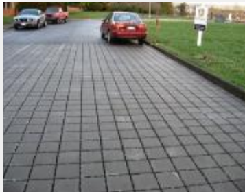
Figure 14. Permeable pavements reduce runoff.
