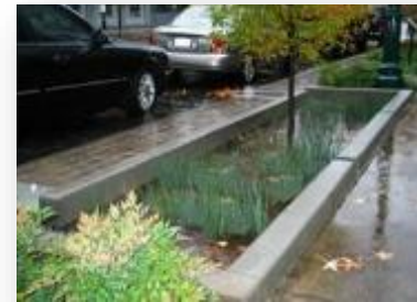
Figure 15. Street planters collect and absorb runoff.
